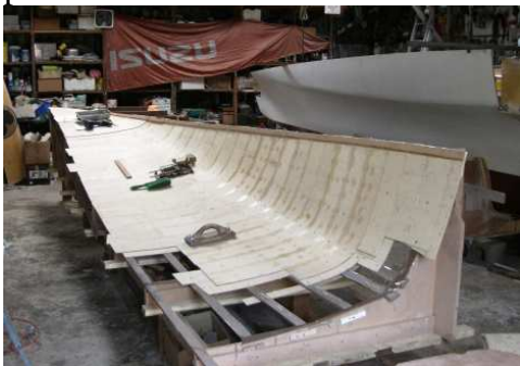
Laminating the half deck
